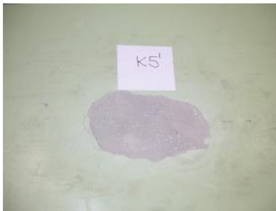
Slika 1. Detalj „otvaranja“ poda usled niskog kvaliteta cementne košuljice Figure 1. The detail of "opening" of the floor due to the low quality cement screed
